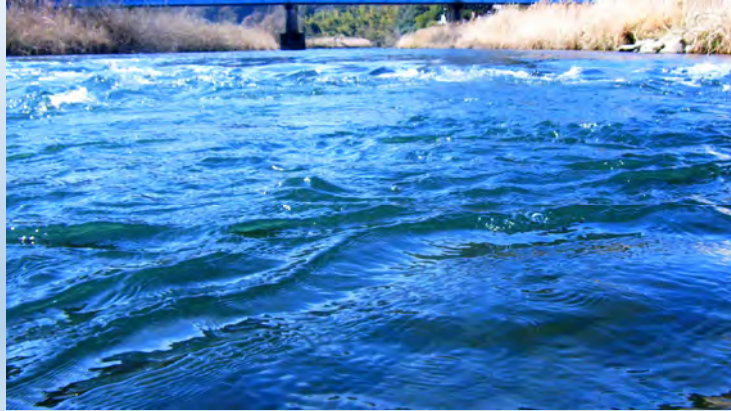
River bed condition after the improvement
