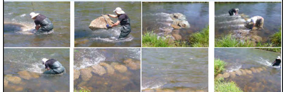
Installation of stacked boulders
